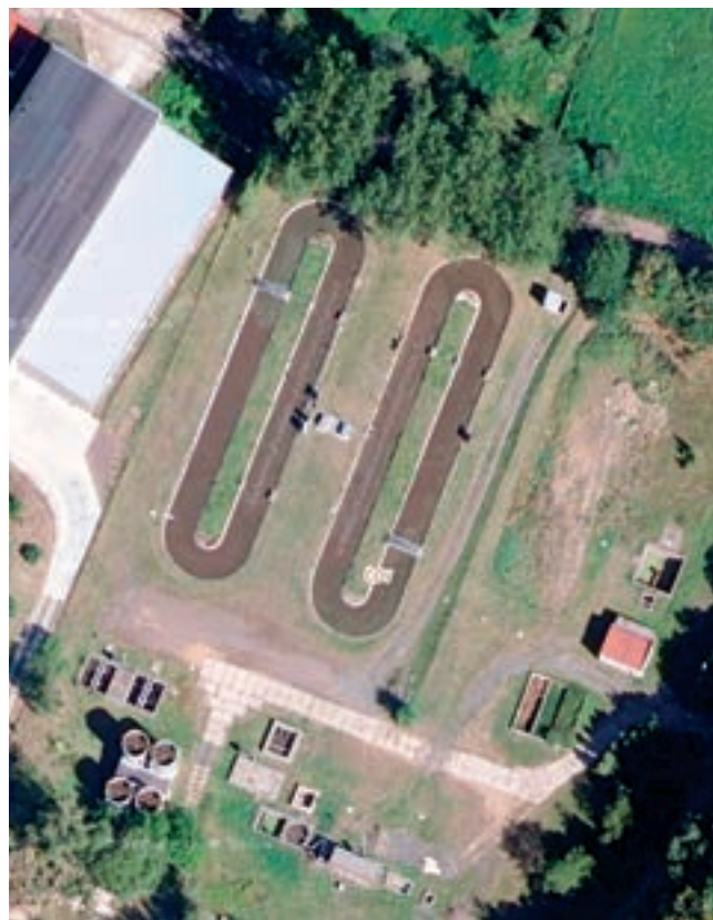
Obr. 3: Areál ČOV Komárov [7]
